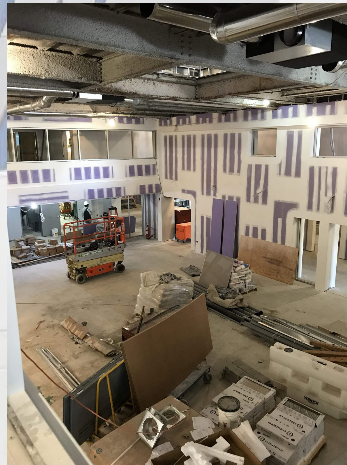
AREA OF MULTI-PURPOSE ROOM 1 AFTER REMOVAL OF 2ND FLOOR SLAB TO CREATE DOUBLE HEIGHT SPACE
