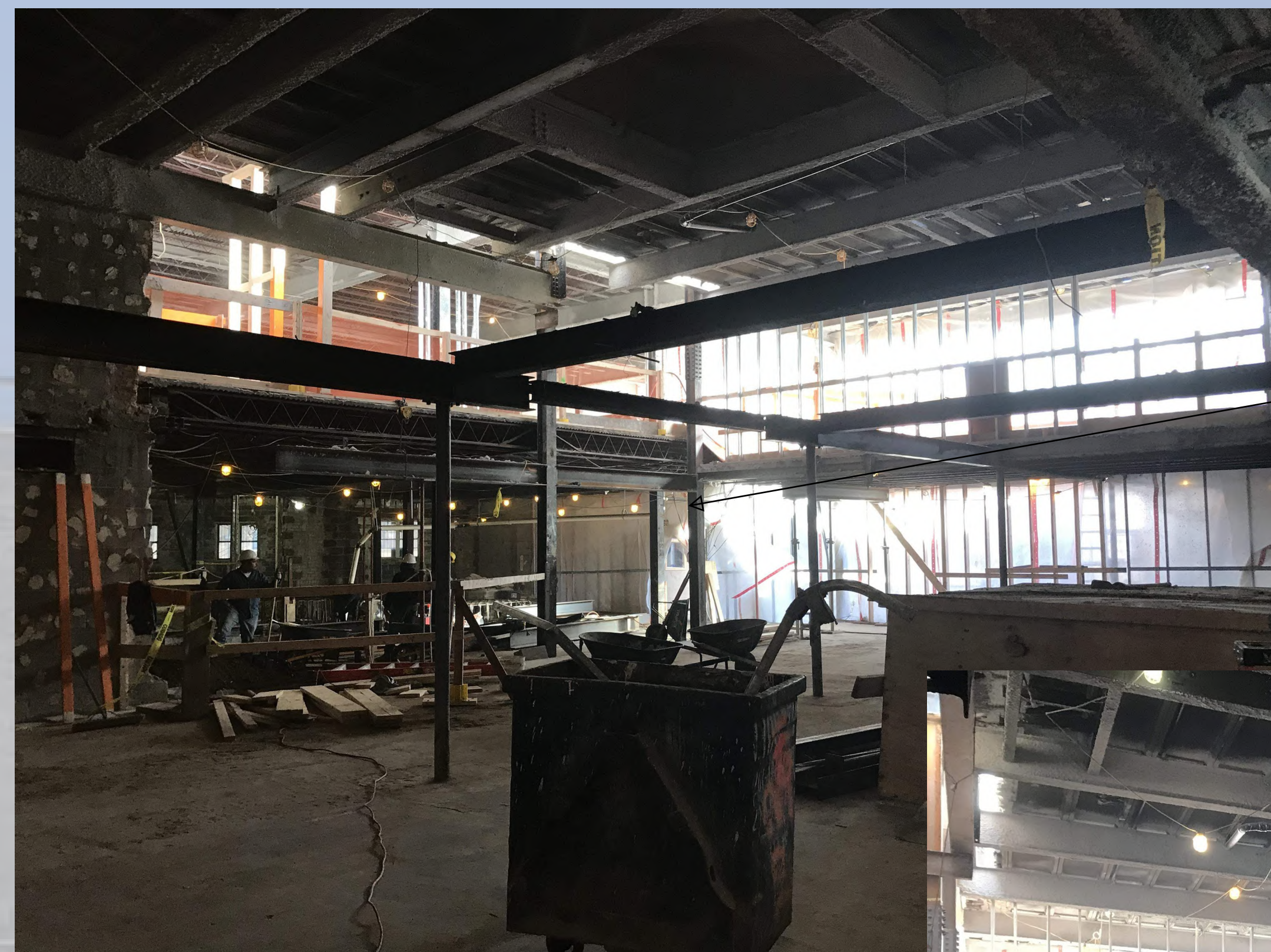
AREA OF MULTI-PURPOSE ROOM 1 AFTER REMOVAL OF 2ND FLOOR SLAB TO CREATE DOUBLE HEIGHT SPACE
